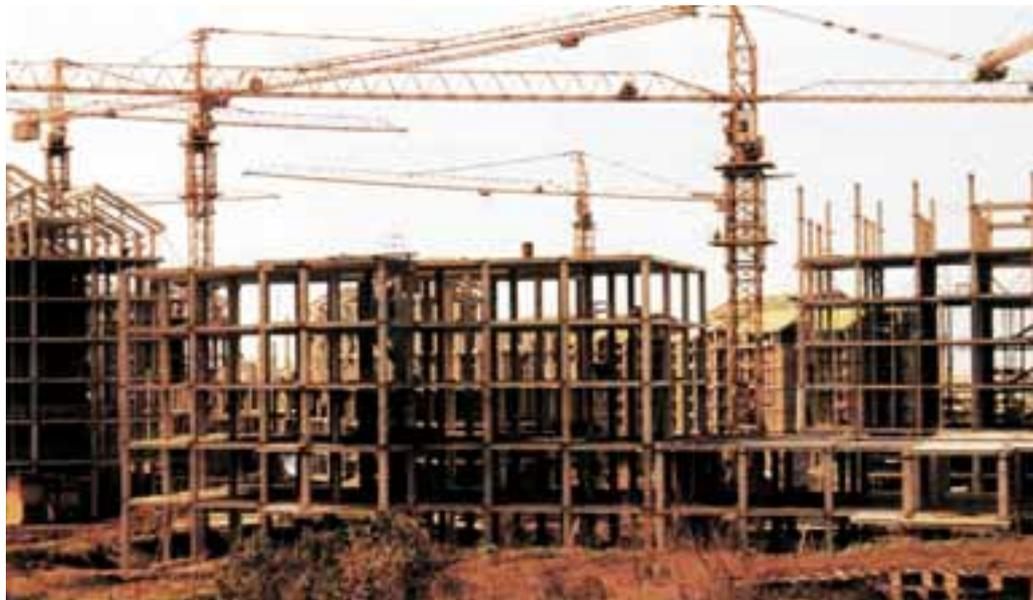
**Defining of** production and assembly process, with adequate norms, enables building control adapted to local conditions, so that appropriate building dynamic is realised and work dead line is reached in time. The IMS Building Technology transfer comprises local labour training for all those processes, with temporary supervision by the IMS Institute experts.
